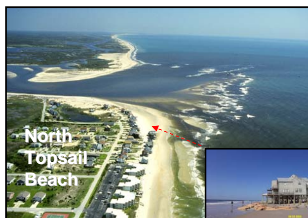
Erosion of oceanfront shoreline related to movement of ebb channel at New River Inlet, NC.
